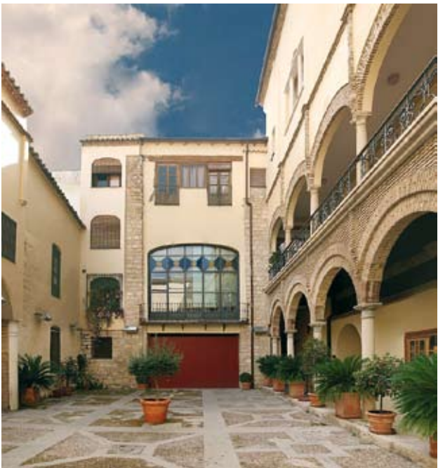
Interior view of the Constable Iranzo's Palace.
